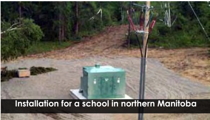
69kV Switch & Fused Pole Structure
