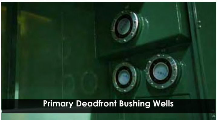
HV Padmount installation for an industrial load
